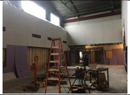
Moisture resistant gypsum board is being installed at areas that are already weathered-in.
