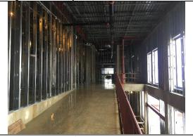
Stud wall framing at  $2^{\text{nd}}$  floor. Interior concrete ramp and stairs.
