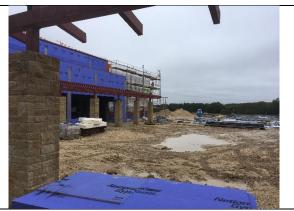
Courtyard View to the Gymnasium. Exterior wall sheathing and masonry columns
